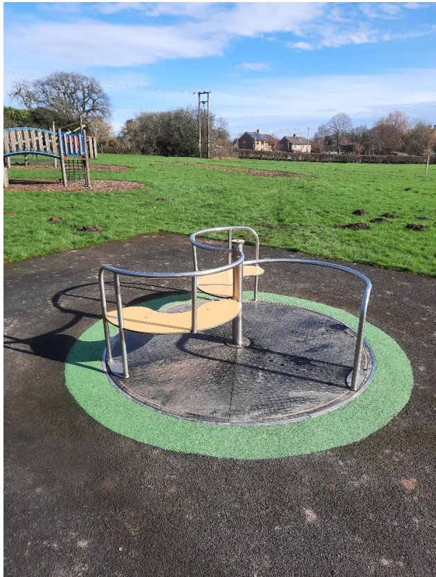
View of repair made to a large 'pot hole' in the roundabout surround in Cuckney Play Park
